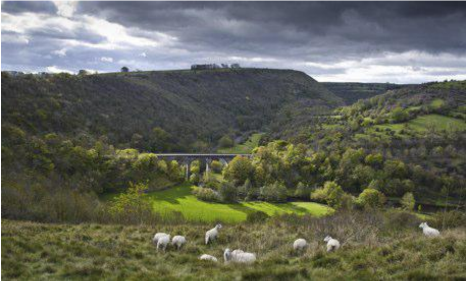
Viaduct over the River
