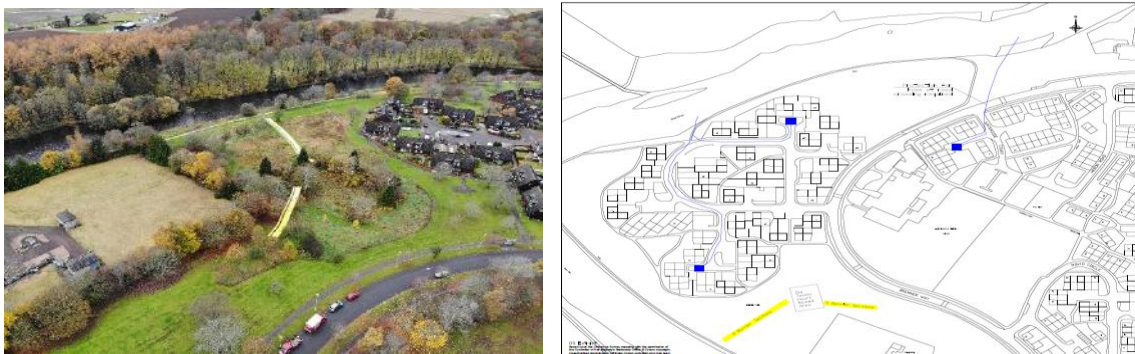
Figure 1: Watergate aerial view & map showing location of pumps: Credit Briggs Marine Services
