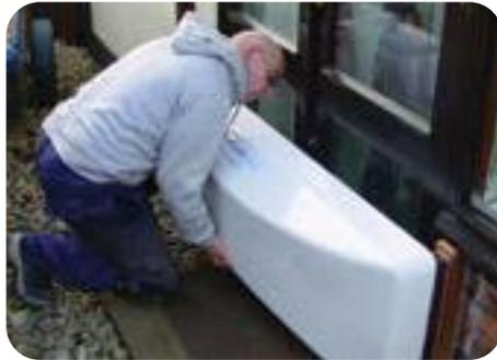
A typical door barrier frame fitted to the exterior brickwork in this case to the main door. Note the frame is fitted to the threshold step, and the subsequent below ground level hole covered with a removable plate. The plate is lifted to gain access to the whole frame in case of a flood situation, the Barrier then being clipped in place.
