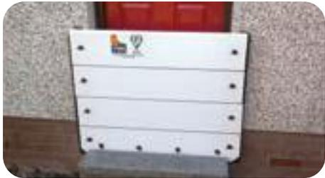
This type of barrier uses a simple clip arrangement to secure it to a preinstalled frame. Each panel is quite light weight and can be used by people who find it difficult to lift heavier objects. This barrier can be used for garage doors as well as other openings. Depending on the property it is not limited to a fixed height of 600 mm as some barriers are – but seek advice first.
