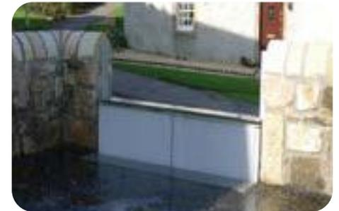
These barriers are quite versatile in that they can be erected and dismantled relatively quickly even able to go around corners. The steel frame is interlinked together and a waterproof sheet is installed over the frame. This is more than sufficient to prevent flood water from reaching critical infrastructure. In this case electrical control equipment. The barriers come in a range of different heights, from 500mm up to 3m.
