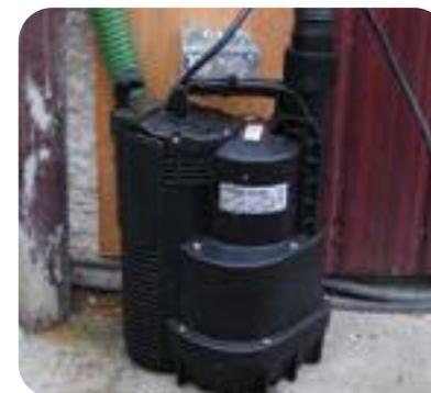
**Sump pumps** – are inexpensive and invaluable in removing water from the solum (under floor void). They can be moved around wherever water may be entering the property. When pumps are fitted to the solum and the water activated, float switch allows the pump to remove water as soon as it reaches a fixed depth. Always use your pump with a RCB safety switch, beware water and electricity are dangerous. We suggest a pump capacity of 500 ltr per min.
