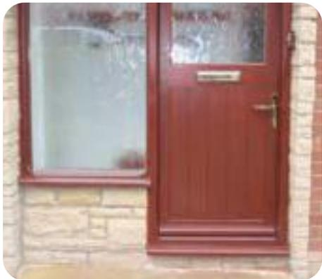
This water proof door is designed and manufactured with a special seal between the frame and the door, which effectively prevents water from entering the property.
