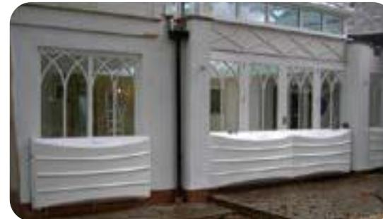
Door barriers can remove much of the worry and fear of flooding. Here a typical door barrier has just been installed – with the property owner within the home, being shown how to fit the barrier in case of a flood. In this case the barrier is installed to the outer brickwork of the property by a permanently fixed frame.
