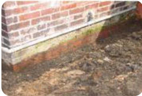
**Persistent damp** – can often be caused by soil piling up against brickwork. This can be through the movement of soil over time. The ideal solution is to cut back soil from the walls of the house and back fill the trench with gravel, this allows surface or ground water to drain away, and prevent water migration up the walls.
