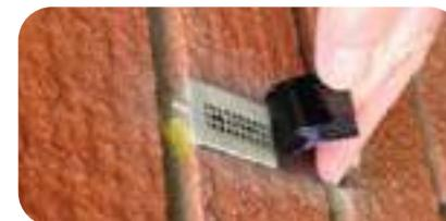
**Micro air vents** – are fitted to many domestic properties throughout Scotland. There are commercially made rubber seals which fit over the vents, however a strip of adhesive flash band obtainable from most DIY shops, and cut to shape will work as well.
