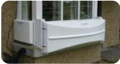
Some door barriers are versatile enough to be used across window openings, where the windows are low enough to be vulnerable to flood risk. In this case the whole estate were equipped with identical products.
