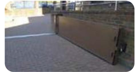
To prevent flood water from affecting a group of houses this water activated hydraulic barrier was installed to a Scottish housing estate. The surrounding walls also act as a flood defence barrier, when lowered the barrier is flush to the ground, when raised the barrier reaches to the top of the wall, about 1m.
