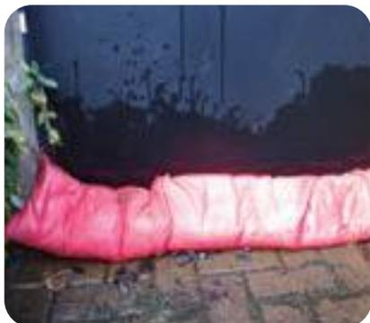
**Synthetic sand bags** – do not contain sand but a special polymer, they are inexpensive and very light unlike sand bags, can be deployed extremely quickly and prevent water from passing through them. They are activated by immersing in water for a few minutes, and molded to fit the location where they are to be used, in this case across a door way and stacked on top of each other up to a height of about 12 – 18 ins. Some can be dried and reused, others are square these here are rectangular.
